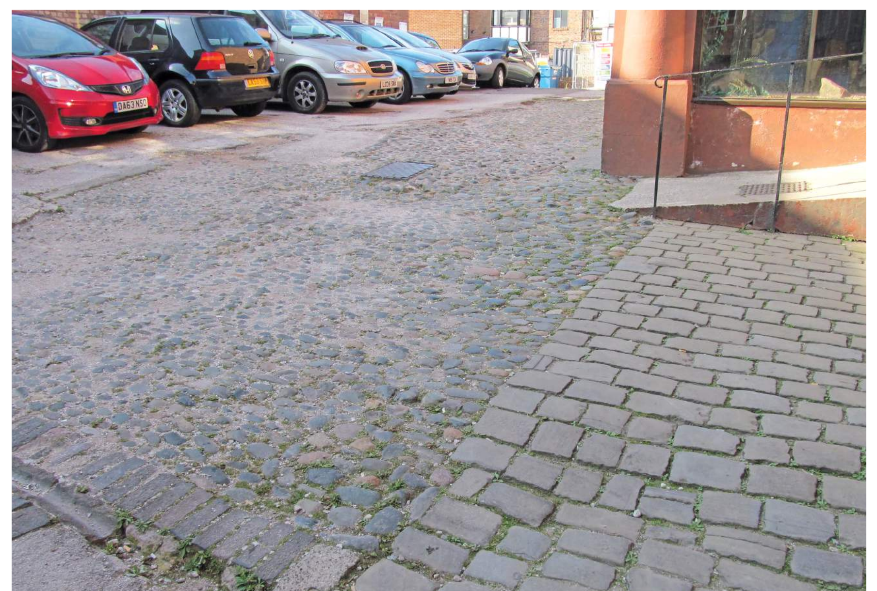
Existing public realm surfacing on Pierpoint Lane needs re-levelling
