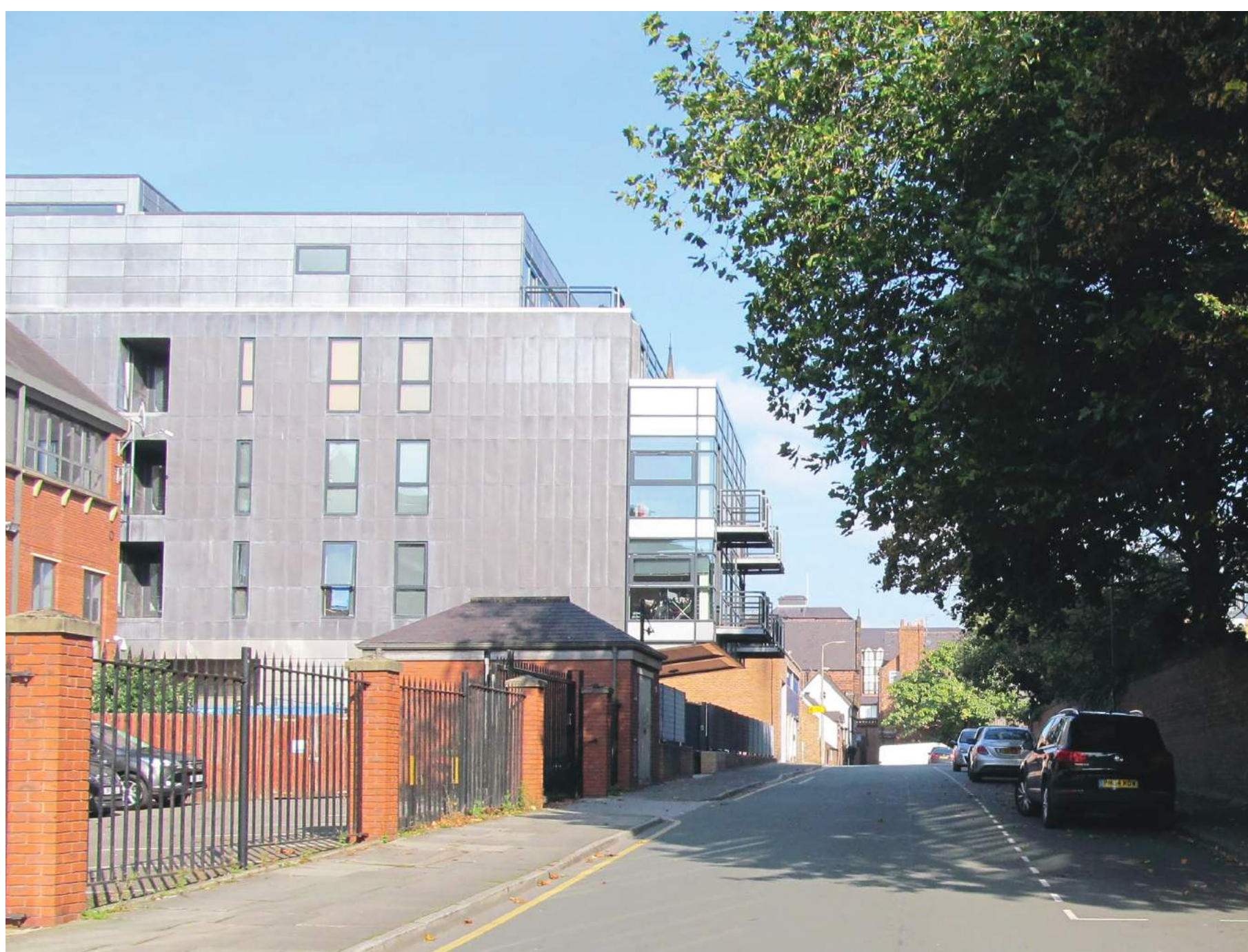
Rear facades of post 1970's development front onto Weaver Street
